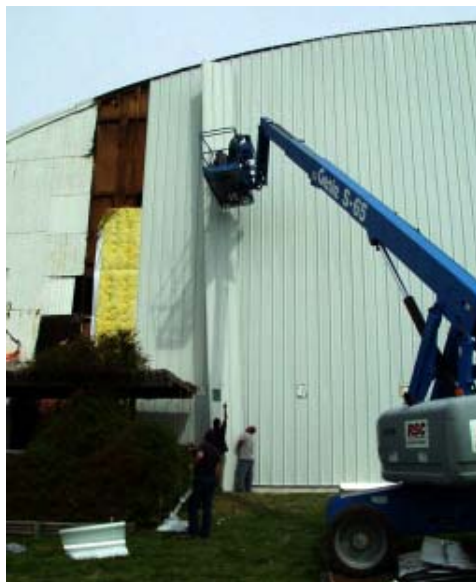
(Far left) Old sheathing is removed from the lean-to. (Center) Old sheathing and plasterboard gone and new insulation going up. (Left) It took a little effort to get a long piece of new sheathing in place. (Below) A new west end for 602.
